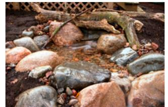
Step 13. With the waterfall running, go around and trim off any excess liner always leaving several inches above the water level/water splash as a precaution. The remaining liner edges can be covered with gravel or other suitable landscape material.
