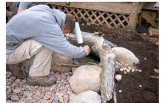
Step 12. Disguising the Waterfall Spillway using boulders, logs, gravel, soil, or other creative landscape material.
