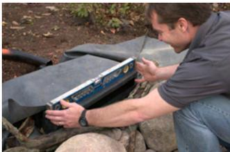
Step 3. Fold liner over top of Waterfall Spillway. It is recommended to provide some slack in the liner in case the position of the Waterfall Spillway needs minor adjustment during installation.
