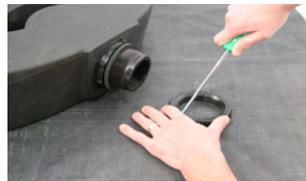
Step 6. Remove the retaining nut and trim a hole in the liner approximately 1/8 inch inside of the score mark.
