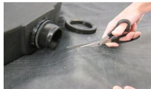
Step 7. Remove the outer rubber gasket from the Waterfall Spillway fitting. Insert the hole in the liner over the Waterfall Spillway fitting. The liner should fit snug around base of the Waterfall Spillway fitting.
