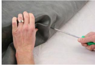
Step 5. Unfold the liner back off the Waterfall Spillway and remove the retaining nut from the Waterfall Spillway fitting. Center the retaining nut over the puncture hole in the liner. Use a pen, marker, or sharp tool, such as an awl or screwdriver to trace a line around the inside of the nut
