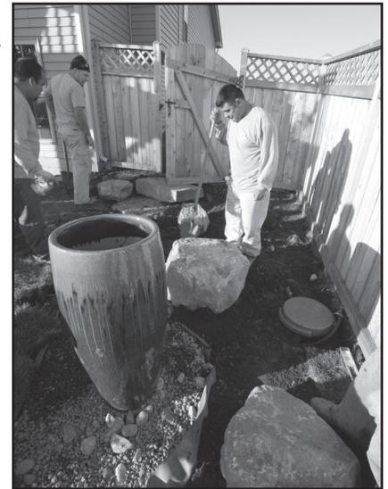
The built-in water level inspection port on the Pondless® Waterfall Vault allows the lid of the Pondless® Waterfall Vault to be buried.
