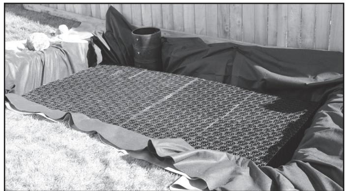
**NOTE:** When stacking AquaBlox® only one panel “A” is required between the two joined AquaBlox®. See tank assembly instructions for more detail.
